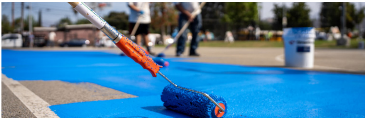
Cool pavement coating installed as part of the GAF Cool Community Project-Pacoima. Credit: Melanie Torres, Pacoima Beautiful.
